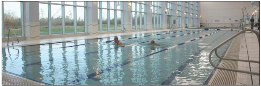
Solar-powered systems heat the water in indoor pools at the Good Shepherd Institute for Healthy Living. Photo: Forbes & Butler. Image courtesy of Good Shepherd Medical Center
