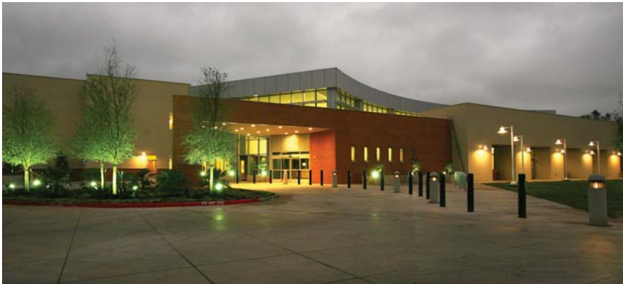
The LEED-certified Good Shepherd Institute for Healthy Living benefits the environment and the health of the region's residents. Photo: Forbes & Butler. Image courtesy of Good Shepherd Medical Center
